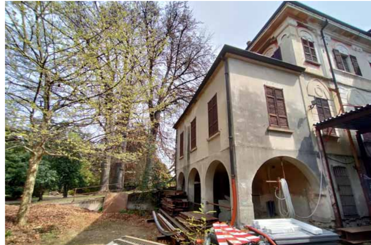
Villa Rossa - North Court
