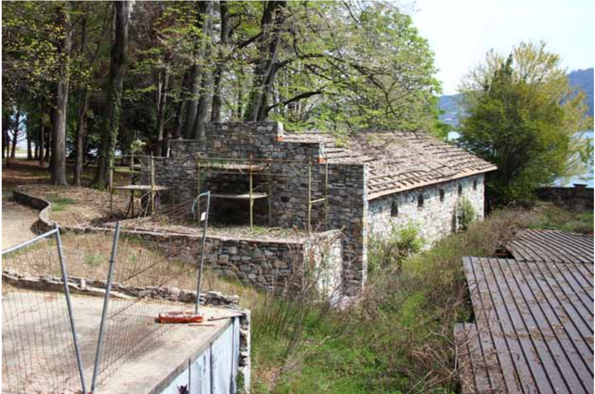
Boat House - Rimessa
